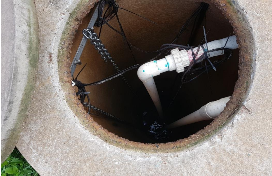
SSP1 Lift well-Inside
