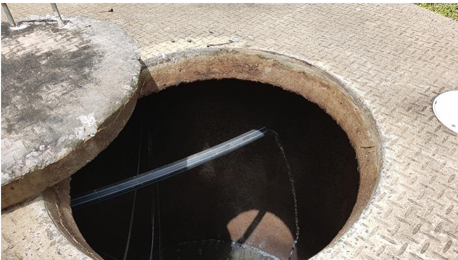
SSP3 Lift Well-Inside
