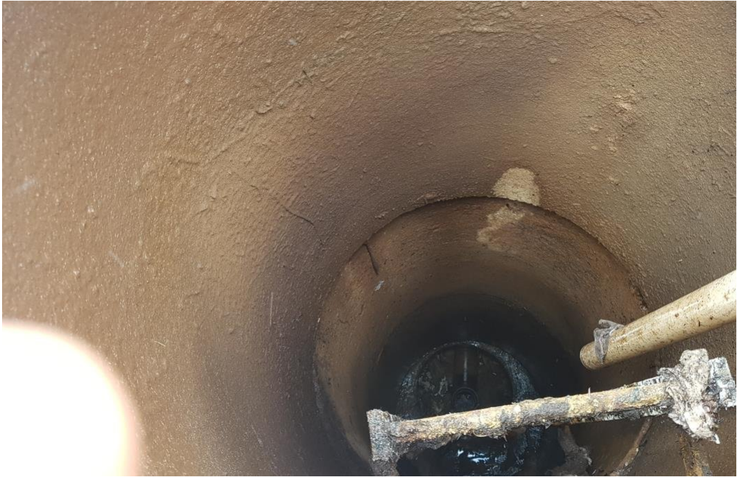
SSP1 Large tank Riser 2 - Inside
