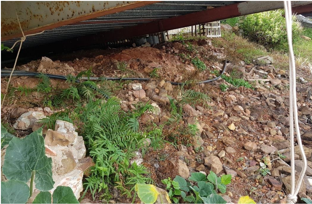
Old SSP3 Discharge Pipe Under Unit 40
